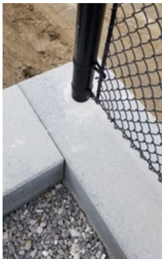
Core Drilled Installation
